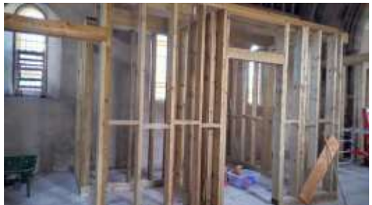
Internal frames for new rooms
