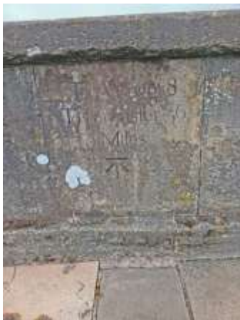
Inscription on downstream parapet of Green Bridge
